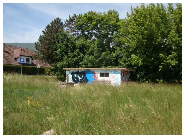
Station de pompage
