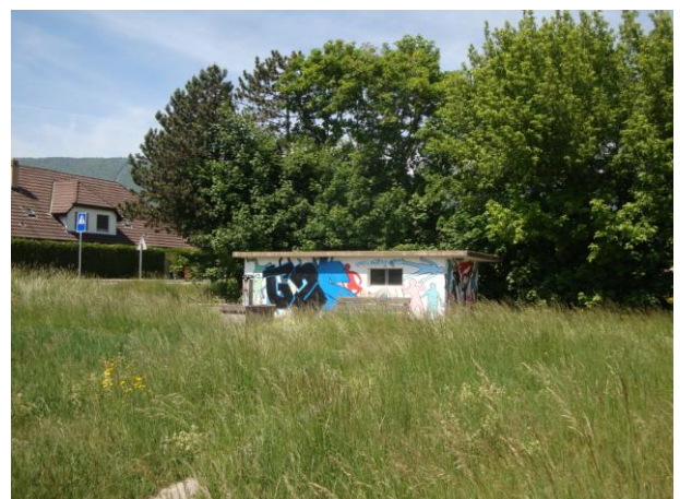
Station de pompage
